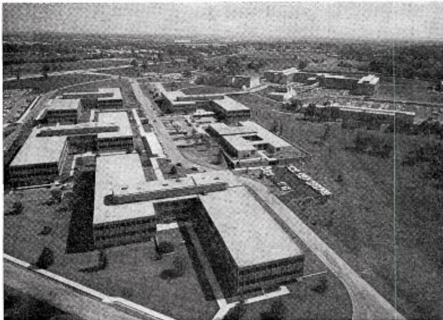
Monsanto Chemical Company's world headquarters in suburban St. Louis is laid out like a modern university. Headquarters of each of Monsanto's
